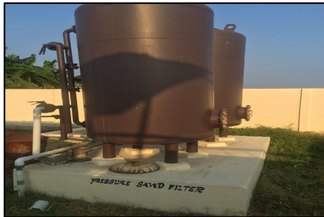
PRESSURE SAND FILTER
